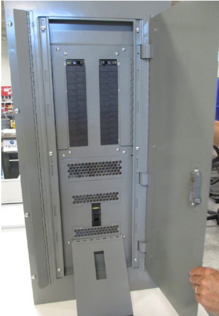
Replacement of Dead Front Panel With Custom Windows
